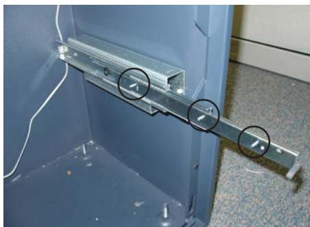
Figure 2. Locking slide rail.
