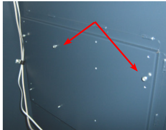
Mounting screws, nuts installed
