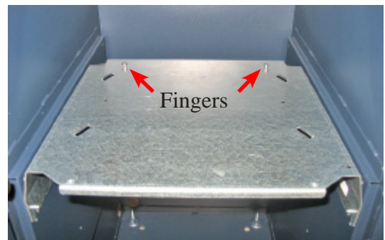
Bracket mounted to cabinet.
