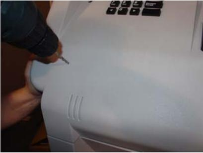
*Figure 4. Drill pilot hole.*
