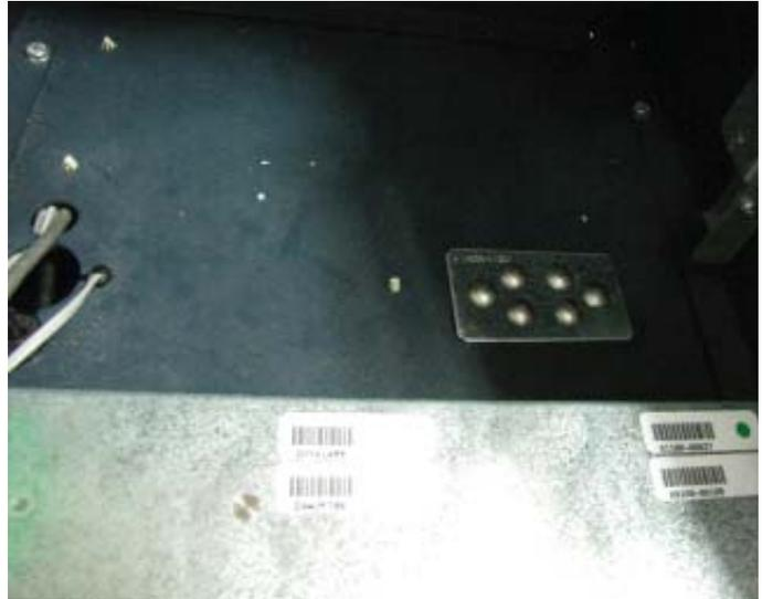
9. Ensure the bolts are not intertwined in the cables in the lower cabinet.
