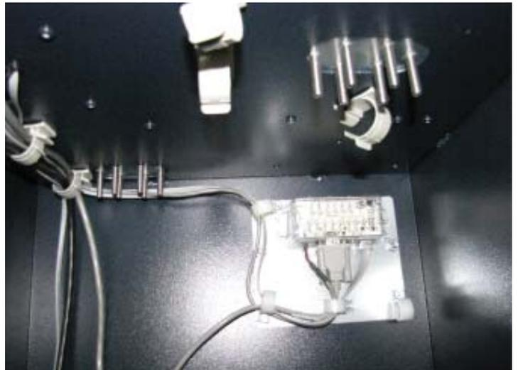
10. Remove the cable clip in the rear left corner of the lower cabinet for easier installation of the closeout bracket.
