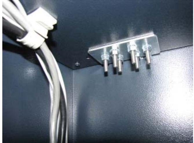
12. Reinstall the cable clip over the closeout bracket as shown.
