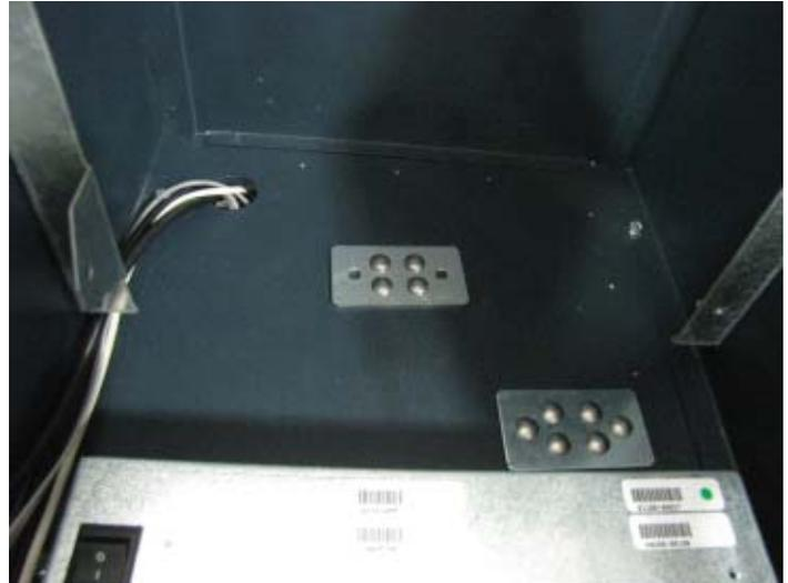
9. Install the lower closeout bracket on the 6 bolts on the right opening. Using the 7/16" hollow shaft but driver, install 6 hex nuts on the bolts. Install the second closeout bracket onto the 4 bolts on the middle opening. Install 4 hex nuts on the bolts. While tightening, ensure the bolts and brackets are sitting flat in the upper cabinet.
