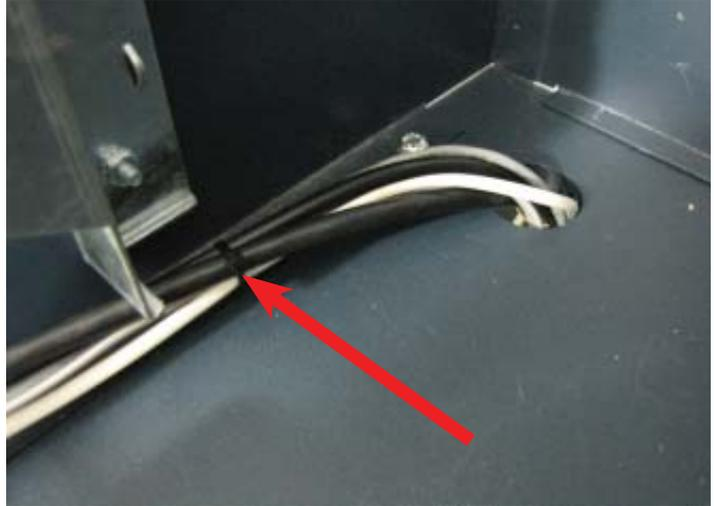
12. Loop the security module power cable back on itself to condense the length of the cable. TY Wrap the cable and cut off the excess.
