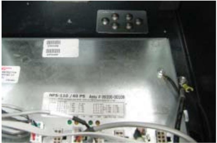
9. Install 4 bolts into one closeout bracket. Set the closeout bracket into the middle circle opening as shown. Ensure the bolts and bracket are sitting flat on the upper cabinet.
