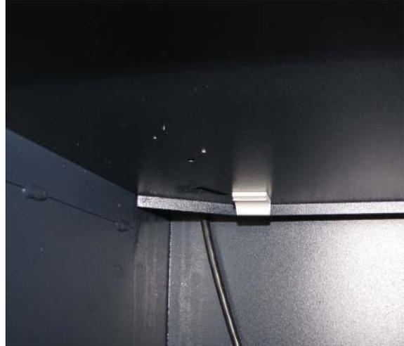
6. Run the data cable over the front of the Mini Mech Tray, then through Adhesive Cable Clip under the tray.
