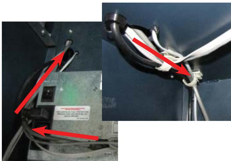
7. Loop the SDD dispenser communication cable back on itself twice to condense the length of the cable to match the length of the dispenser power cable. TY Wrap the two cables together in two spots as shown. Cut off the excess TY Wraps.
