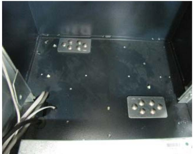
10. Ensure the bolts are not intertwined in the cables in the lower cabinet. Remove the cable clip from the rear left of the lower cabinet.
