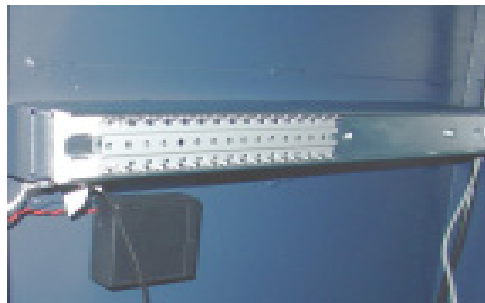
Slide rail installed. (representative)
